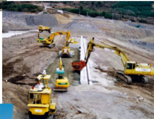
Placing of concretes
