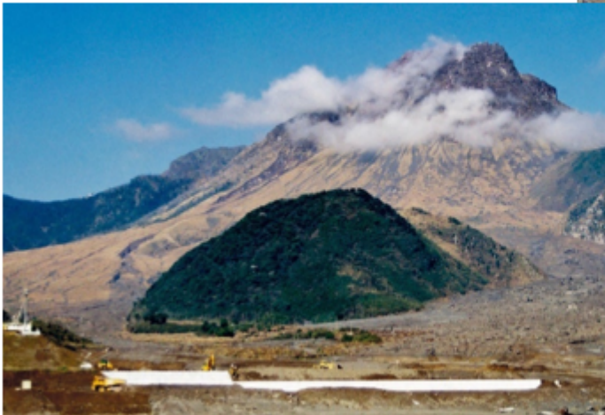
Overall view of completed block setting
