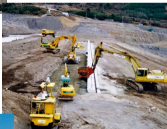
Placing of concretes
