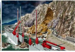
works on the top of pile wall, it minimises working space down to just contacted area of piles on the ground and eliminates a need for temporary platform even on slope, unlevelled ground and above water.
