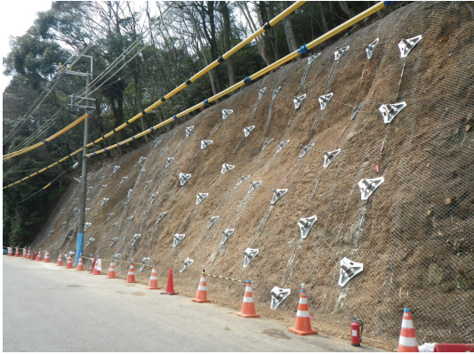
Right after construction of NONFRAME® method
