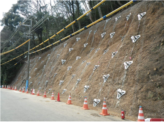
Right after construction of NONFRAME® method
