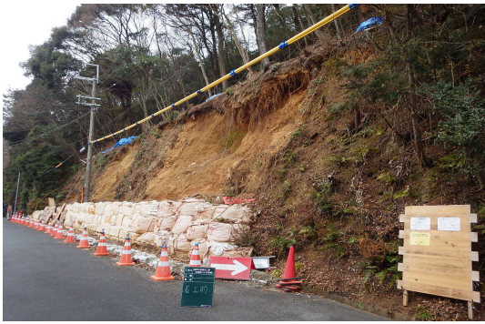
Right after slope failure
