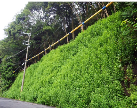
4 months after construction, the slope had been fully covered
