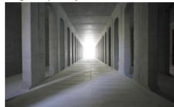
[Example: Box culvert tank, Storage capacity 4,400 m<sup>3</sup>]
