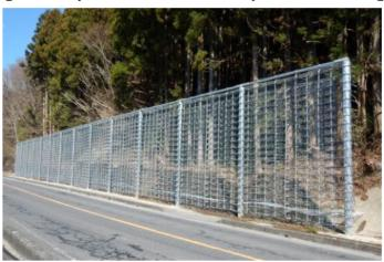
【Example: Shallow Landslide protection, with Finished Paint】
