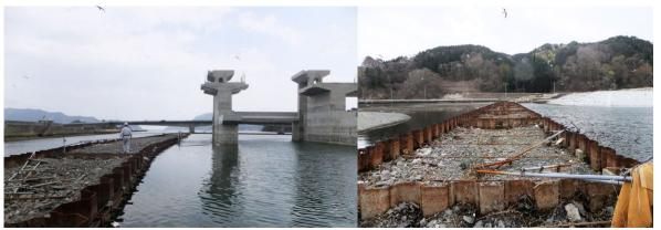
At the time of the Great East Japan Earthquake, a similar structure was adopted as a temporary cofferdam structure for the construction of a tide gate near the river mouth of the Iwakasa River in Iwate Prefecture. While the surrounding river embankments and the residential area were destroyed, double steel sheet pile walls and the floodgates built inside the cofferdam were almost free from the tsunami damage, demonstrating their high earthquake resistance and tsunami resistance.
