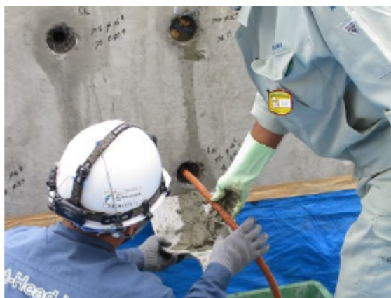
③ Mortar filling
