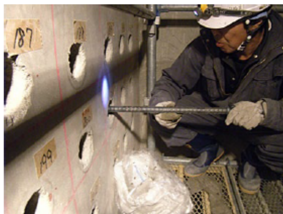
④ Inserting PHbs
